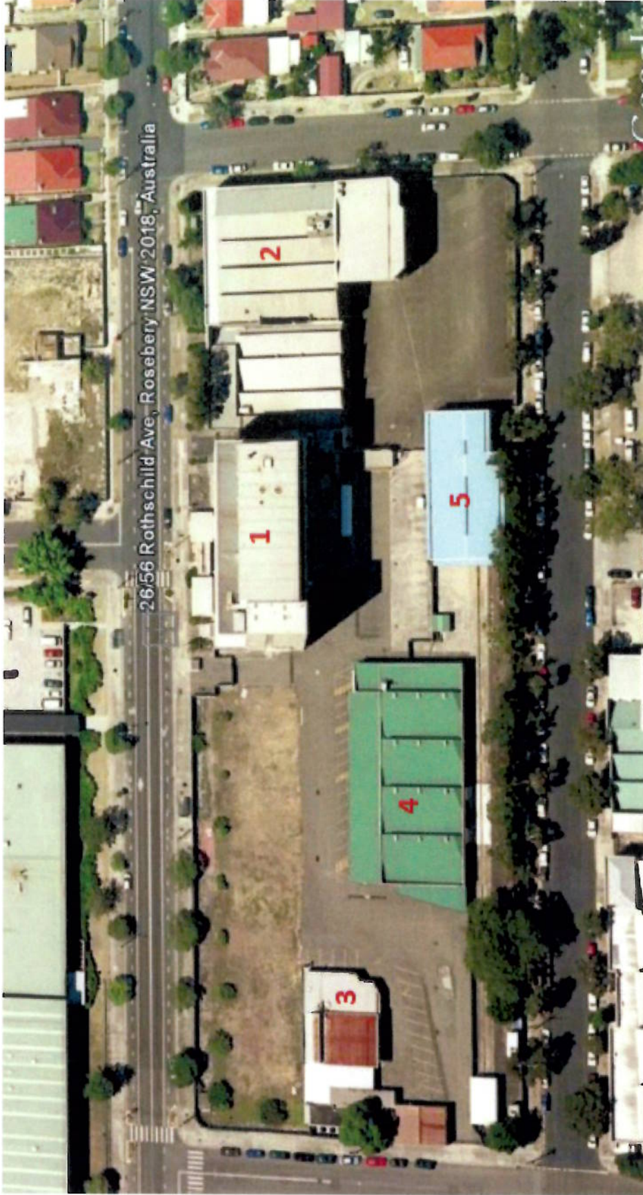
Photo of existing Buildings to be demolished
